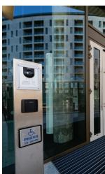
An RFID tag is installed in a key card or fob which building occupants use to access the building. RFID readers are installed near the door to which they manage access. These readers are fitted with antennas that receive the data transmitted by the RFID tags.
